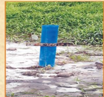
DIGGING OF BOREWELLS
