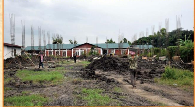
ONGOING CONSTRUCTION OF GIRLS' HOSTEL
